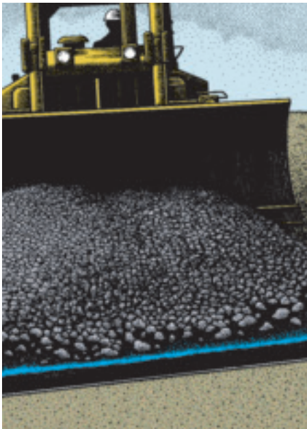
Propex heavyweight nonwoven geotextiles allow the construction of landfill drainage layers without fear of liner damage.
