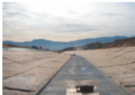
Installation of Pyramat high performance turf reinforcement mat (HPTRM) on this drainage channel in Mesquite, Nevada was specified because of the product's superior UV resistance, high tensile strength, and overall durability.
