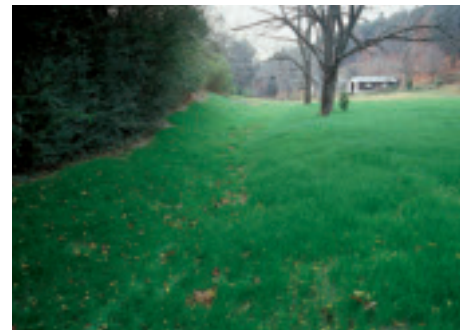
As the ECB degrades, vegetation prevents sediment runoff. The channel now blends nicely with its environment.
