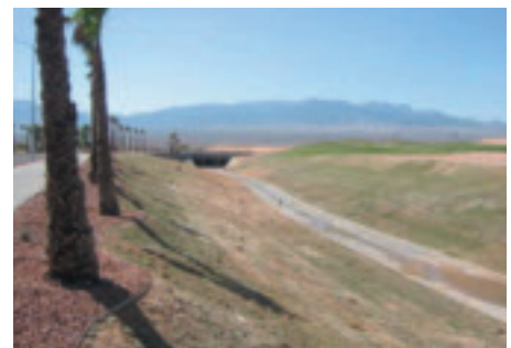
Installation of Pyramat high performance turf reinforcement mat (HPTRM) on this drainage channel in Mesquite, Nevada was specified because of the product's superior UV resistance, high tensile strength, and overall durability.
